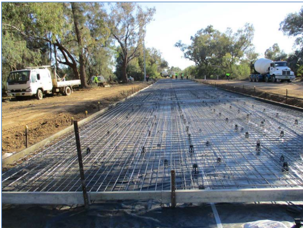
Photo 6: Construction of a new concrete causeway on Watercourse Road
